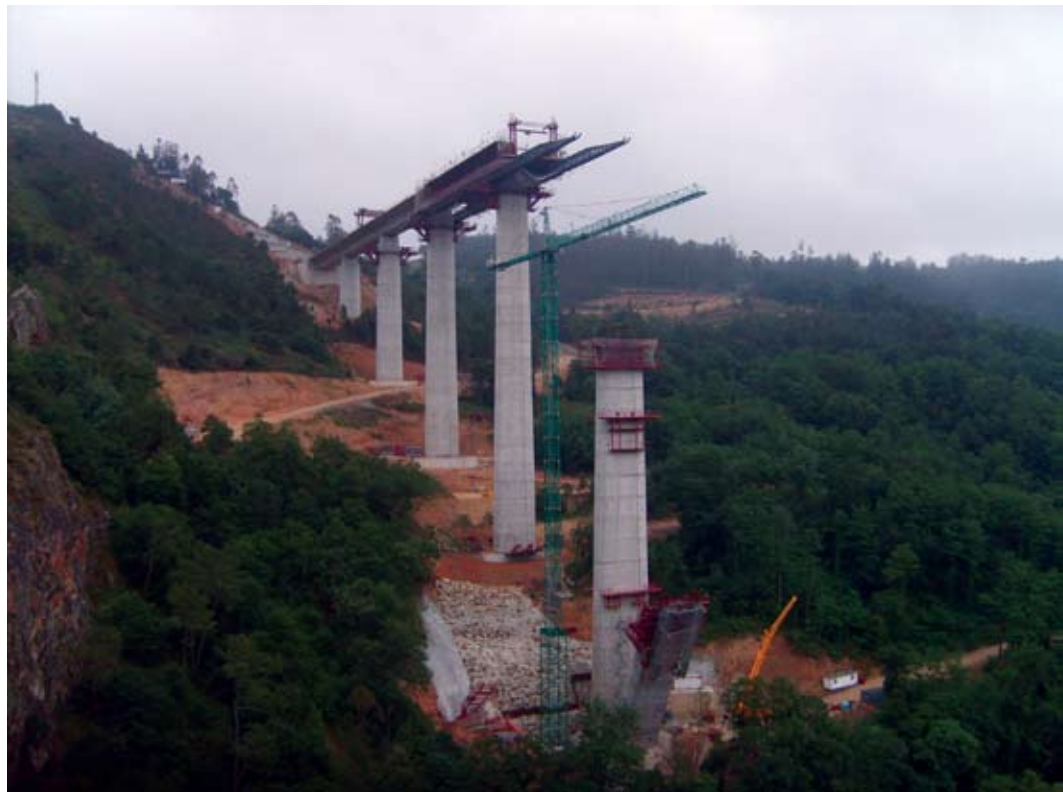
Construction of high-speed rail lines in other countries has created thousands of jobs. Here, construction is underway on a bridge as part of Spain's efforts to extend its high-speed rail network. Credit: Xosema, used under Creative Commons license
